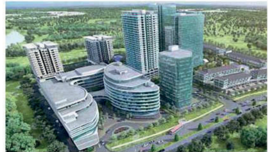
Kerjaya Prospek Group Bhd's Edusphere @ Cyberjaya project. Up to end-November, Kerjaya Prospek had secured about RM1.5 billion in new contracts, boosting its outstanding order book to RM4.1 billion.
